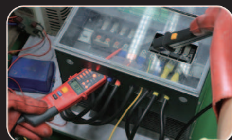
Phase rotation test
